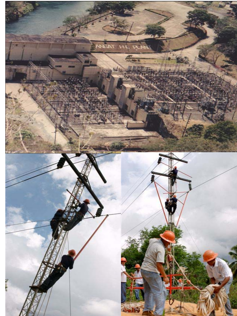
Top photo shows the Angat hydroelectric power plant. Below, technical crew undertakes maintenance and upgrading operations for the transmission lines.
